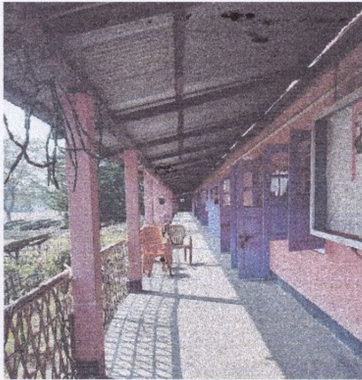
A view of College Verandah
